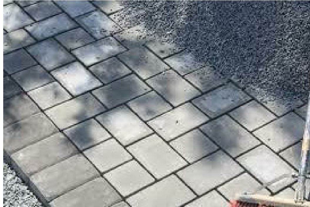
EXTERIOR WALKWAY MATERIAL PERMEABLE PAVERS, TBD
