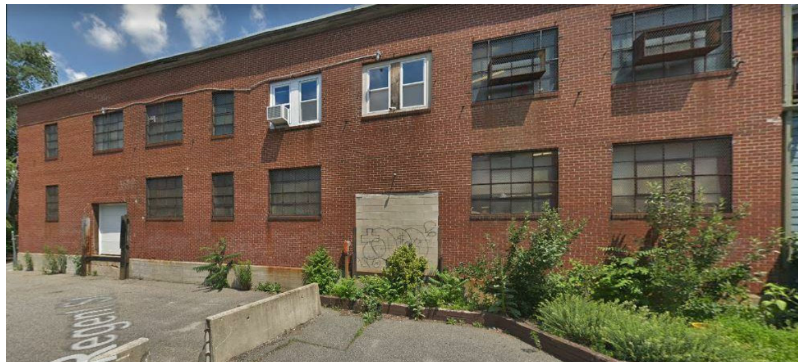
56 CREIGHTON, VIEW FROM TRAIN TRACKS
