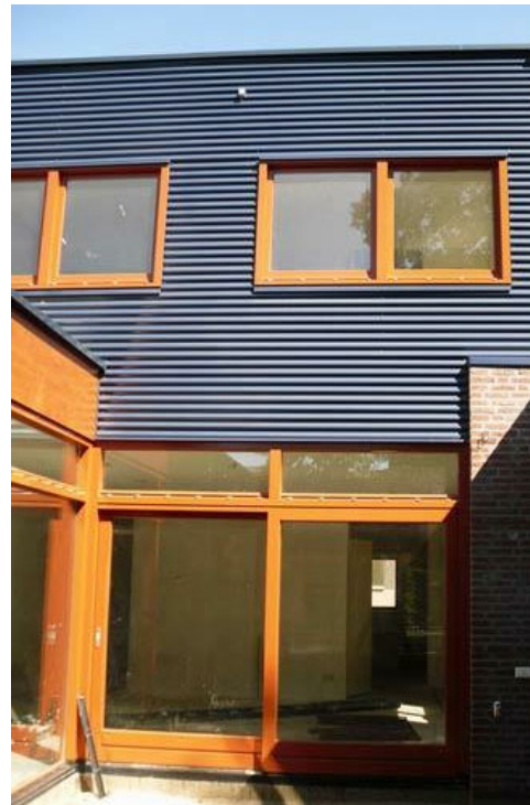
EXTERIOR CLADDING HORIZONTAL METAL SIDING, TBD
