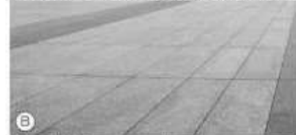
B Granite Pavement
