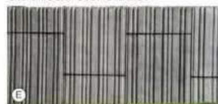
E Formed Concrete Wall
