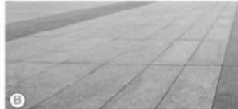
B Granite Pavement
