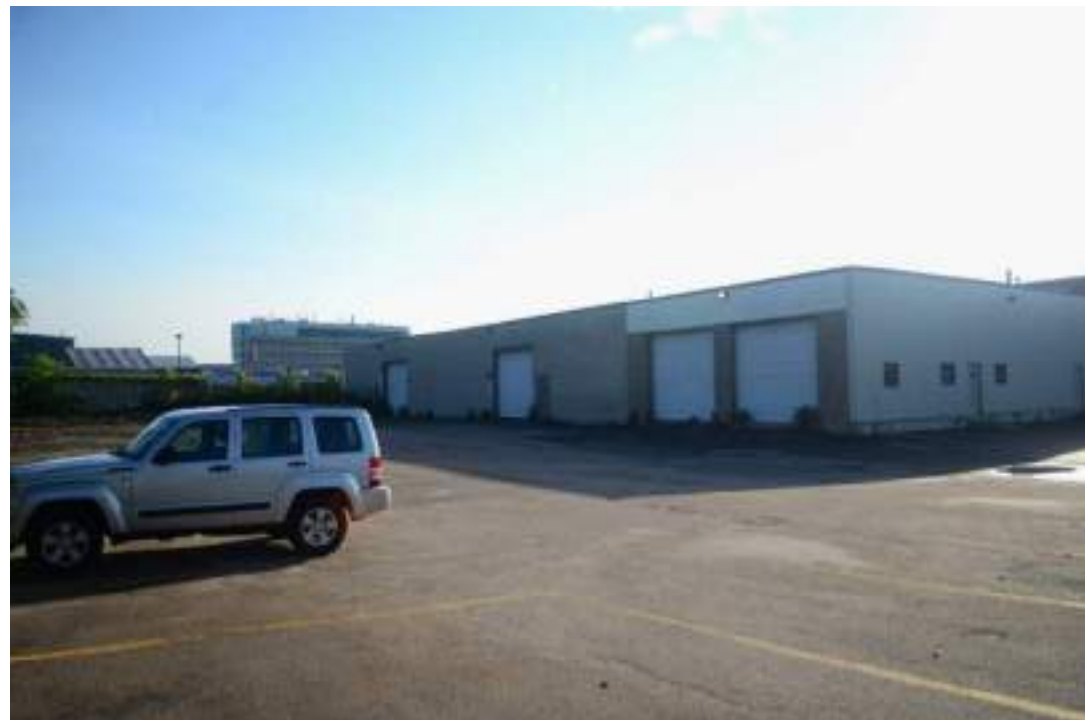
SOUTH WEST: PHOTO FROM ADLEY ROAD, REAR OF SITE 03
