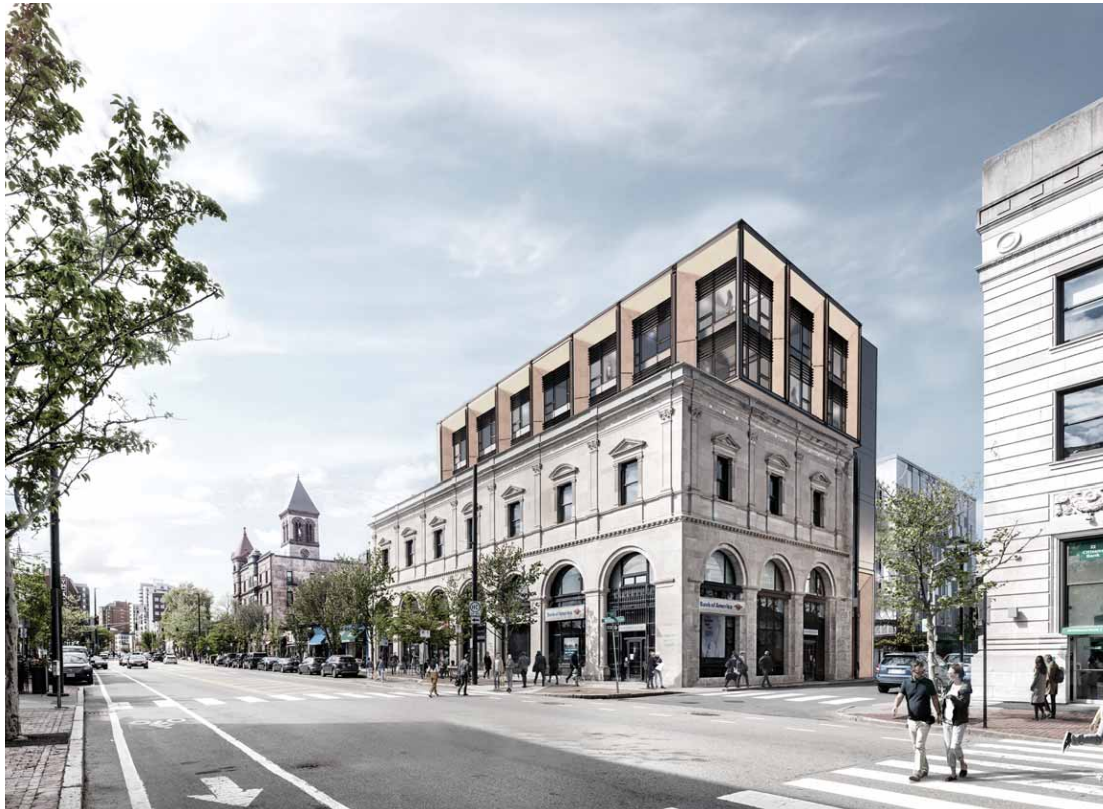
① View from Massachusetts Ave Looking West
