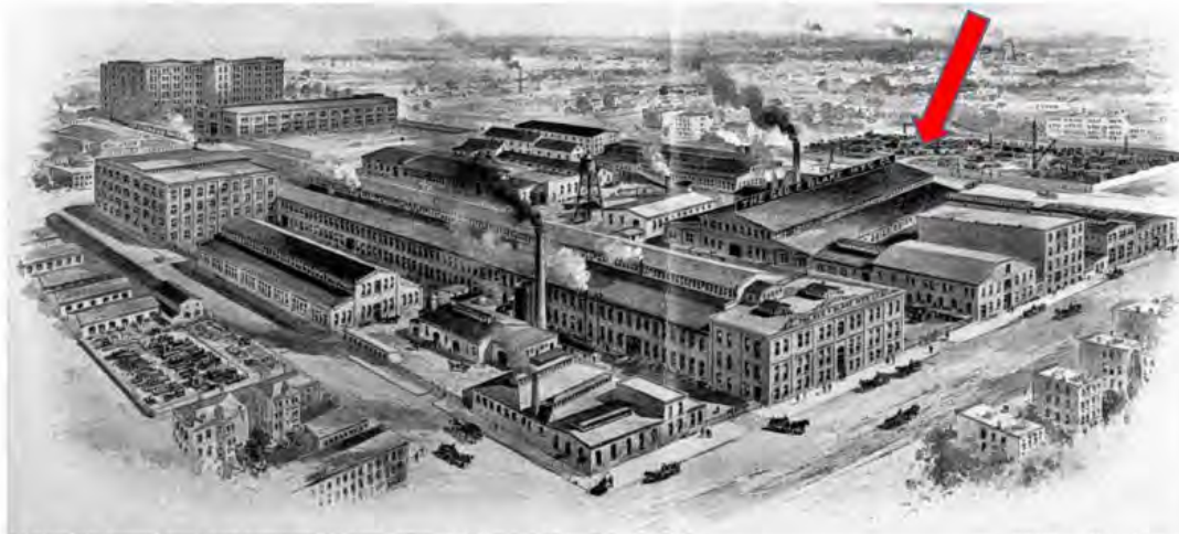
Blake & Knowles Works, ca. 1910. Arrow indicates Foundry Building
