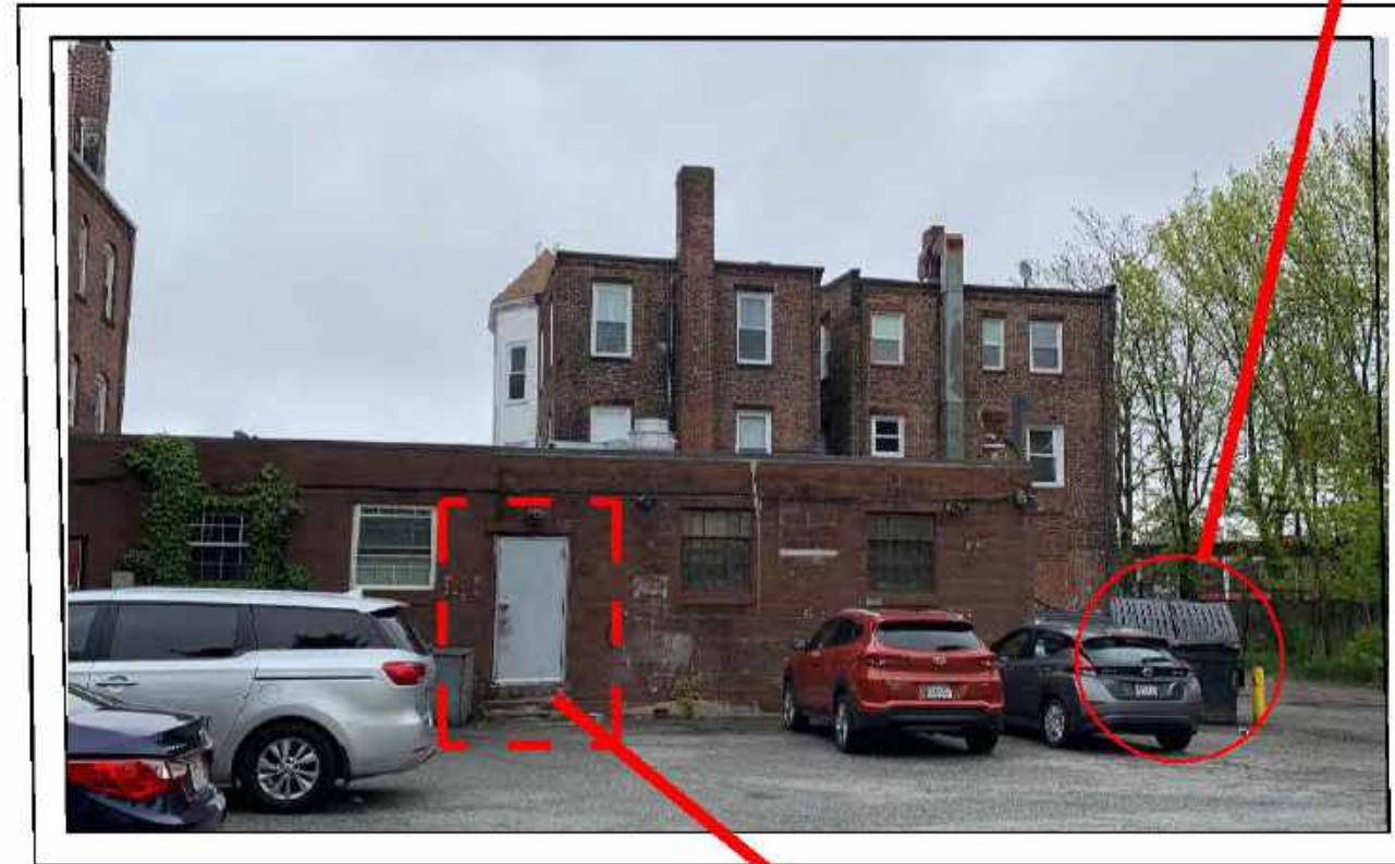
DELIVERY ACCESS (EXISTING) FROM REAR PARKING LOT
