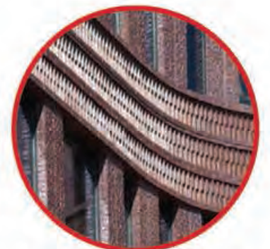
6. HORIZONTAL BRICK BELTS WITH ARTICULATED BRICK DETAILING
