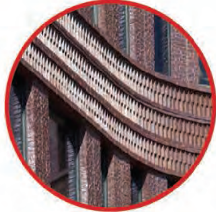
6. HORIZONTAL BRICK BELTS WITH ARTICULATED BRICK DETAILING
