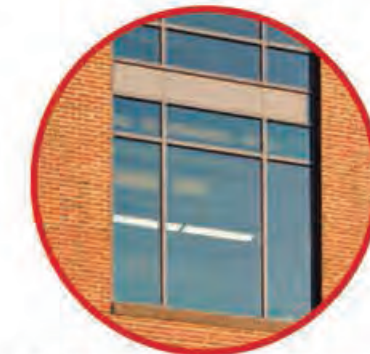
3. VERTICAL BRICK PIERS WITH METAL TRANSOM PANELS
