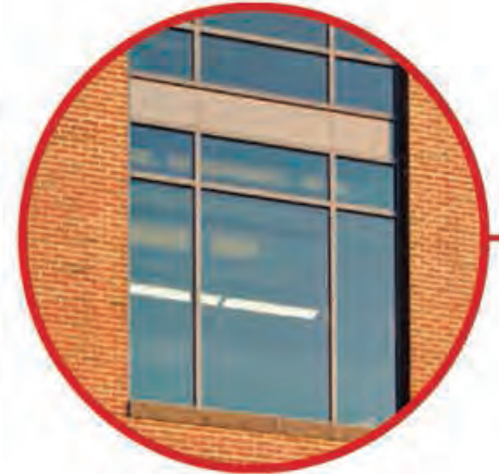
3. VERTICAL BRICK PIERS WITH METAL TRANSOM PANELS
