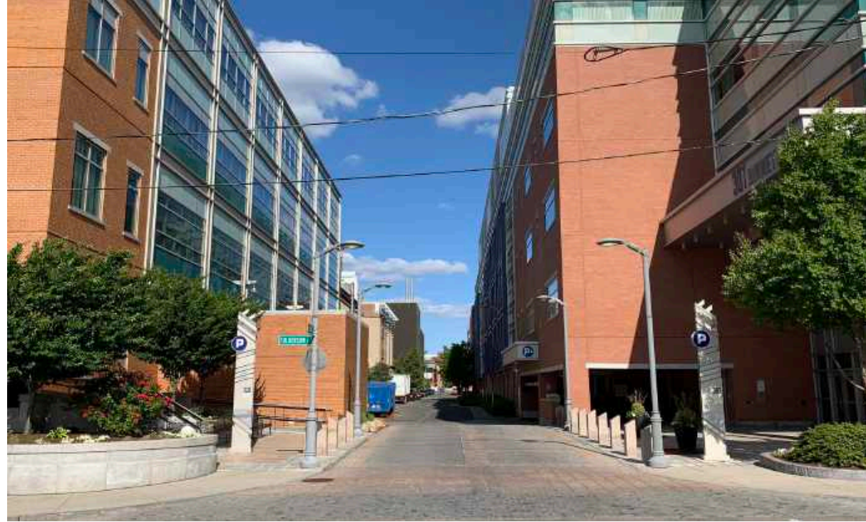
View from Fulkerson Street to Rogers Street, looking East
