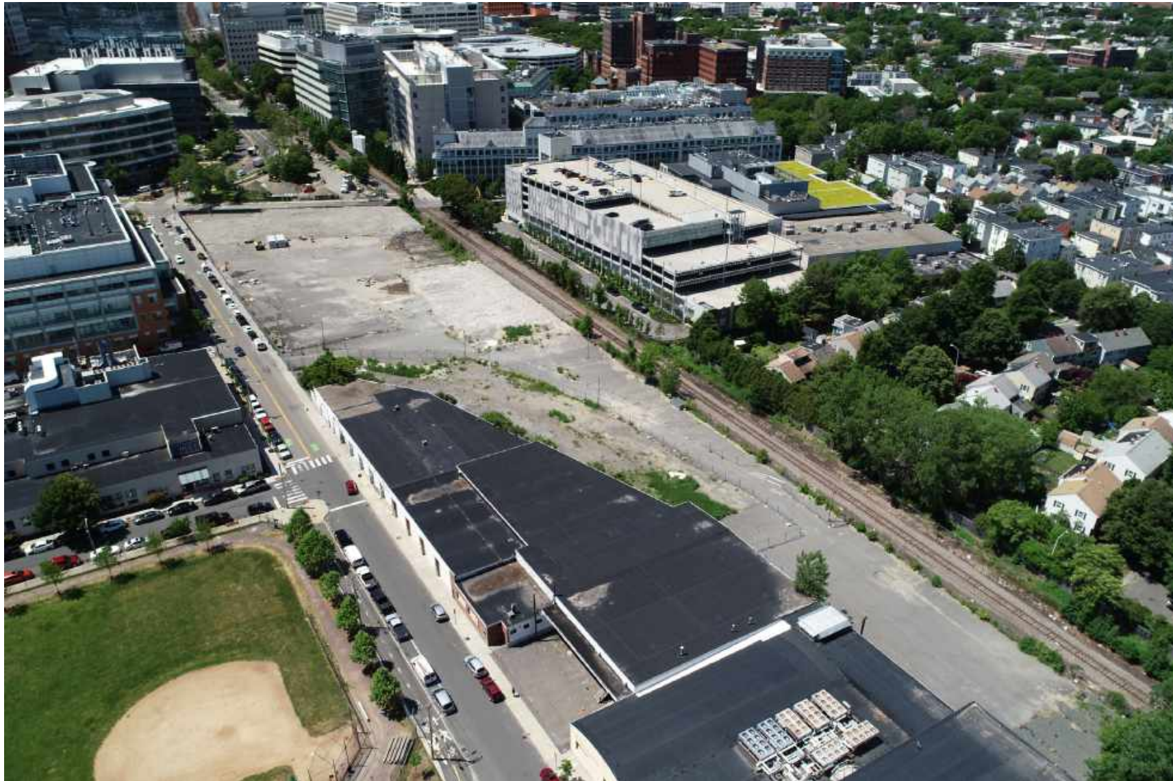
View from Northeast, Looking Southwest
