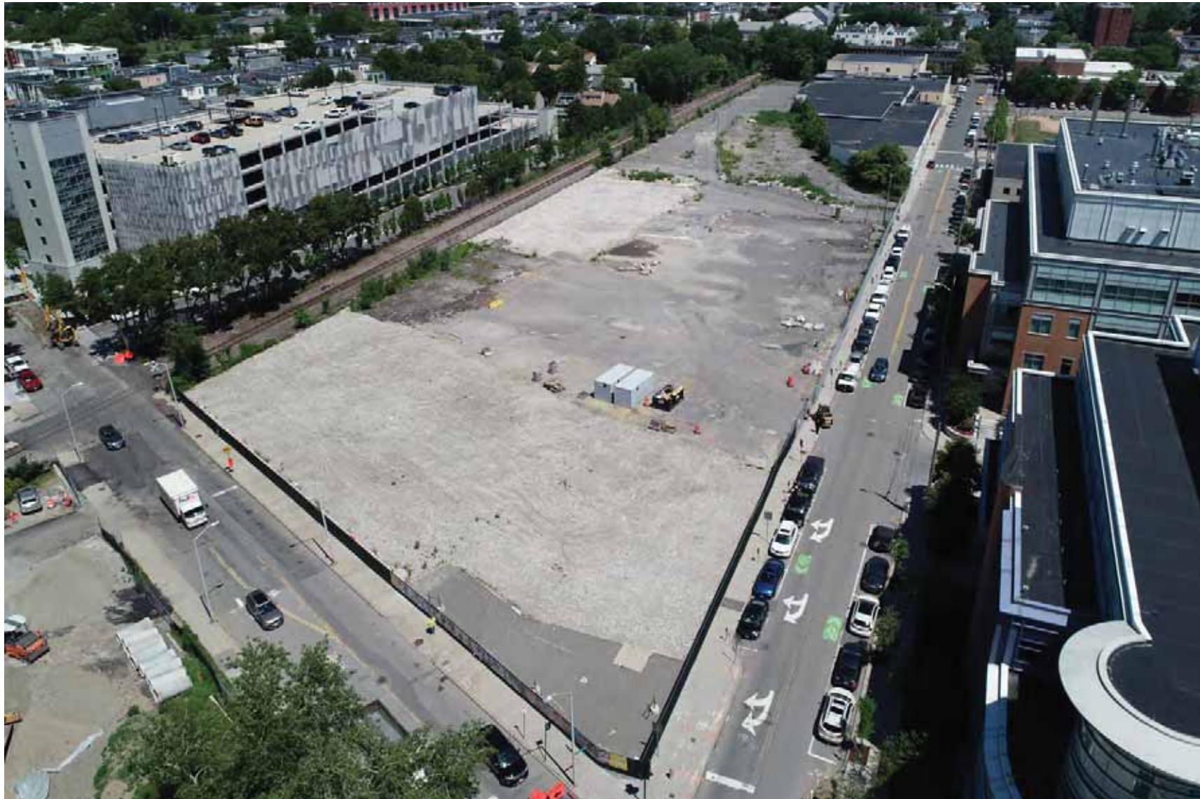
View from South/Southeast, Looking North
