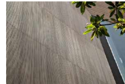
⑨ Custom Finish Metal Panel Soffit to Match Accent Panel Color
