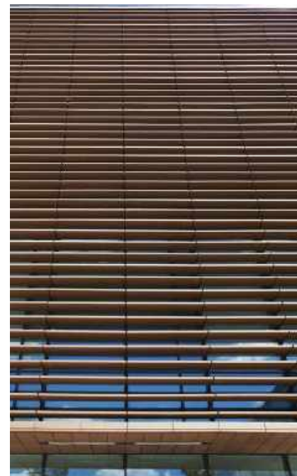
⑧ Integrated Horizontal Sun Shade at Curtain Wall with Ultra High Performance Concrete or Custom Finished Metal to Match Accent Panel Color
