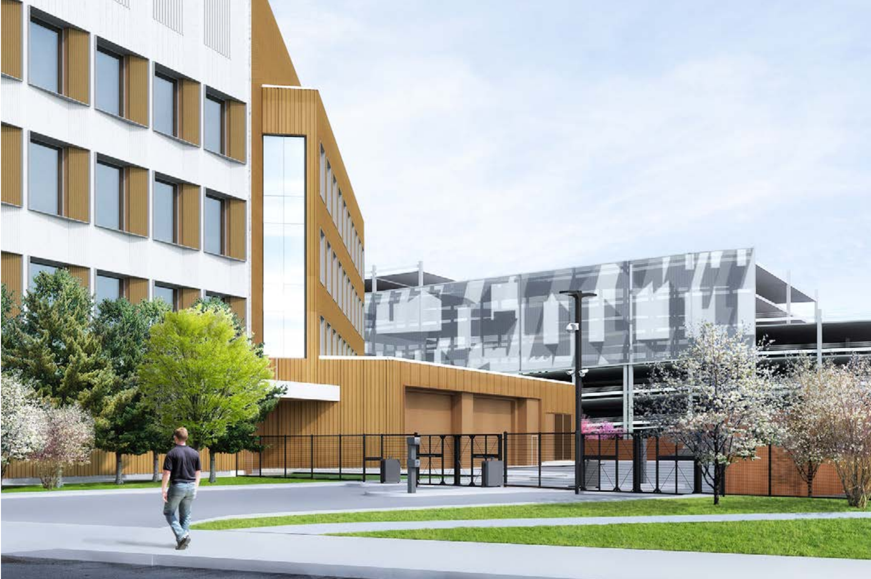
View From Fulkerson Toward Loading Dock Drive and Security Gate (Zoom in)
