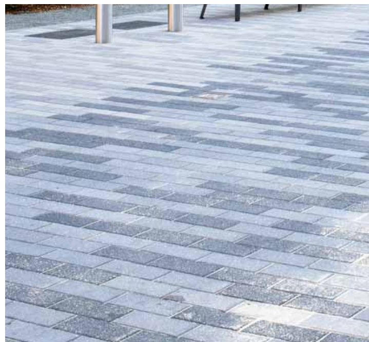
CONCRETE UNIT PAVING
