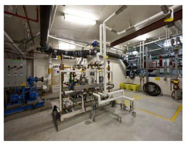
Figure 21. Image of blackwater treatment system in NYC project – Courtesy of Natural Systems Utilities
