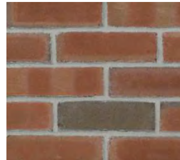
1 REBUILT BRICK WALL @ GREEN ST
