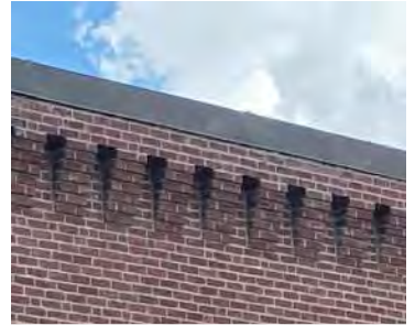
Photo of existing cornice to be rebuilt
