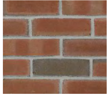
3 REBUILT BRICK WALL @ GREEN ST
