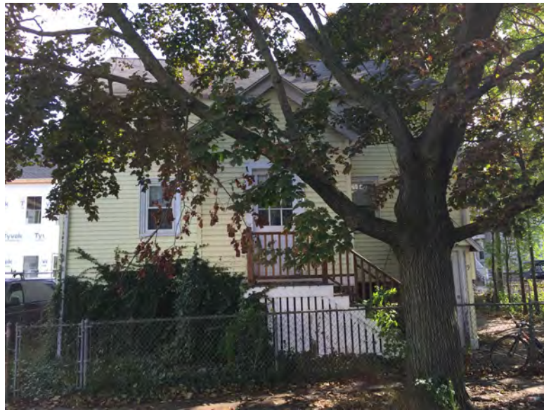
EXISTING JACKSON ST FACADE, WEST ELEVATION
