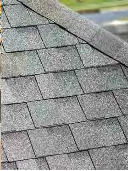
ASPHALT SHINGLE ROOF
