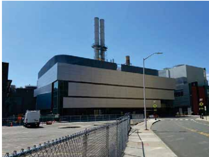
East side of Portland St, looking south towards Albany St
