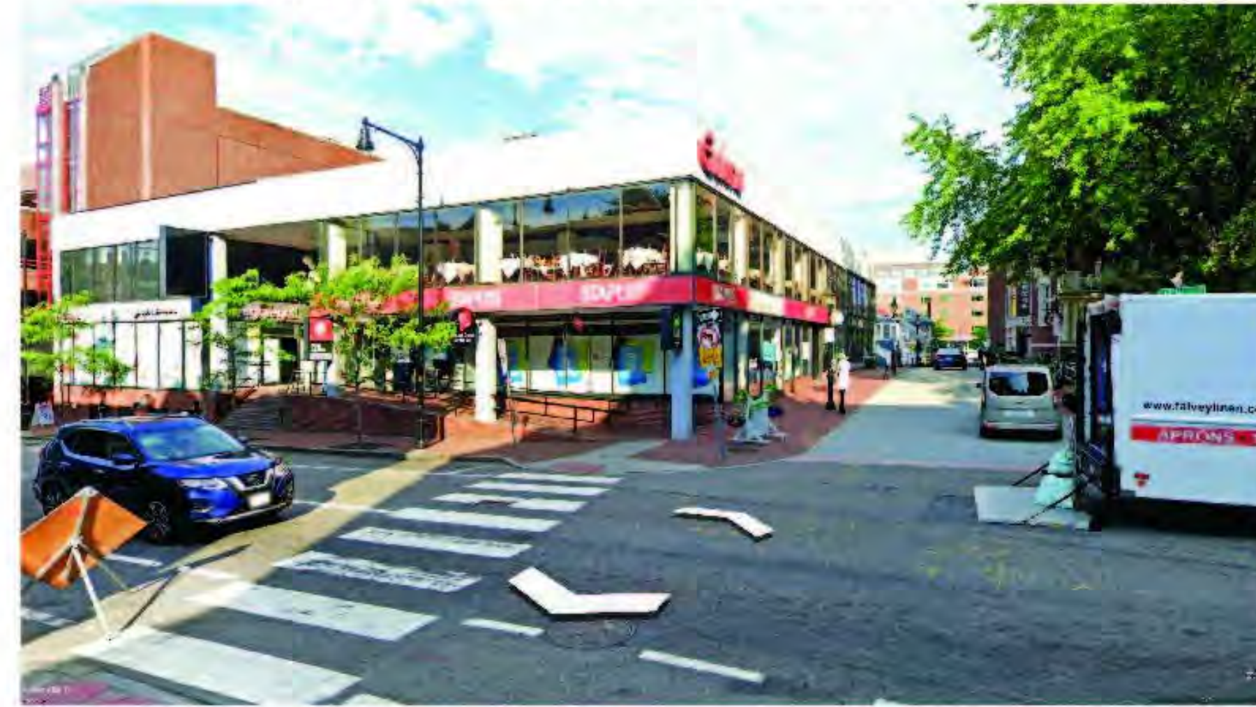
EXISTING EXTERIOR VIEW AT JFK ST
