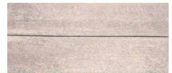
⑥ Concrete Pavement
