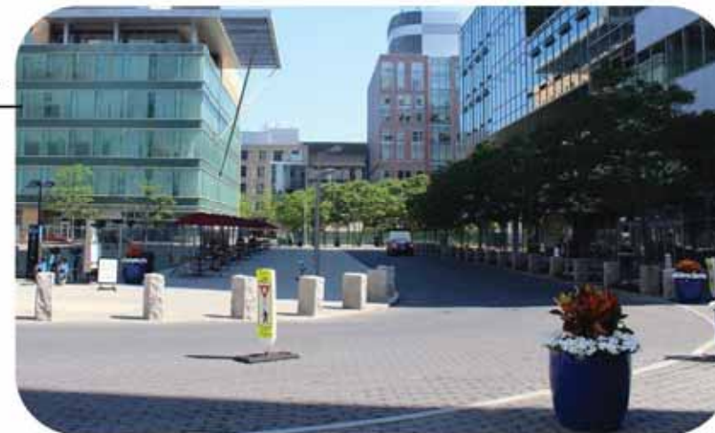
EXISTING KENDALL STREET
