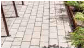
PERMEABLE UNIT PAVERS - TYPE 2
