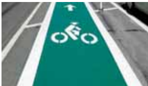
PERMEABLE ASPHALT BIKE PATH
