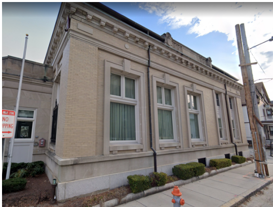
Existing Southwest Façade Treatment
