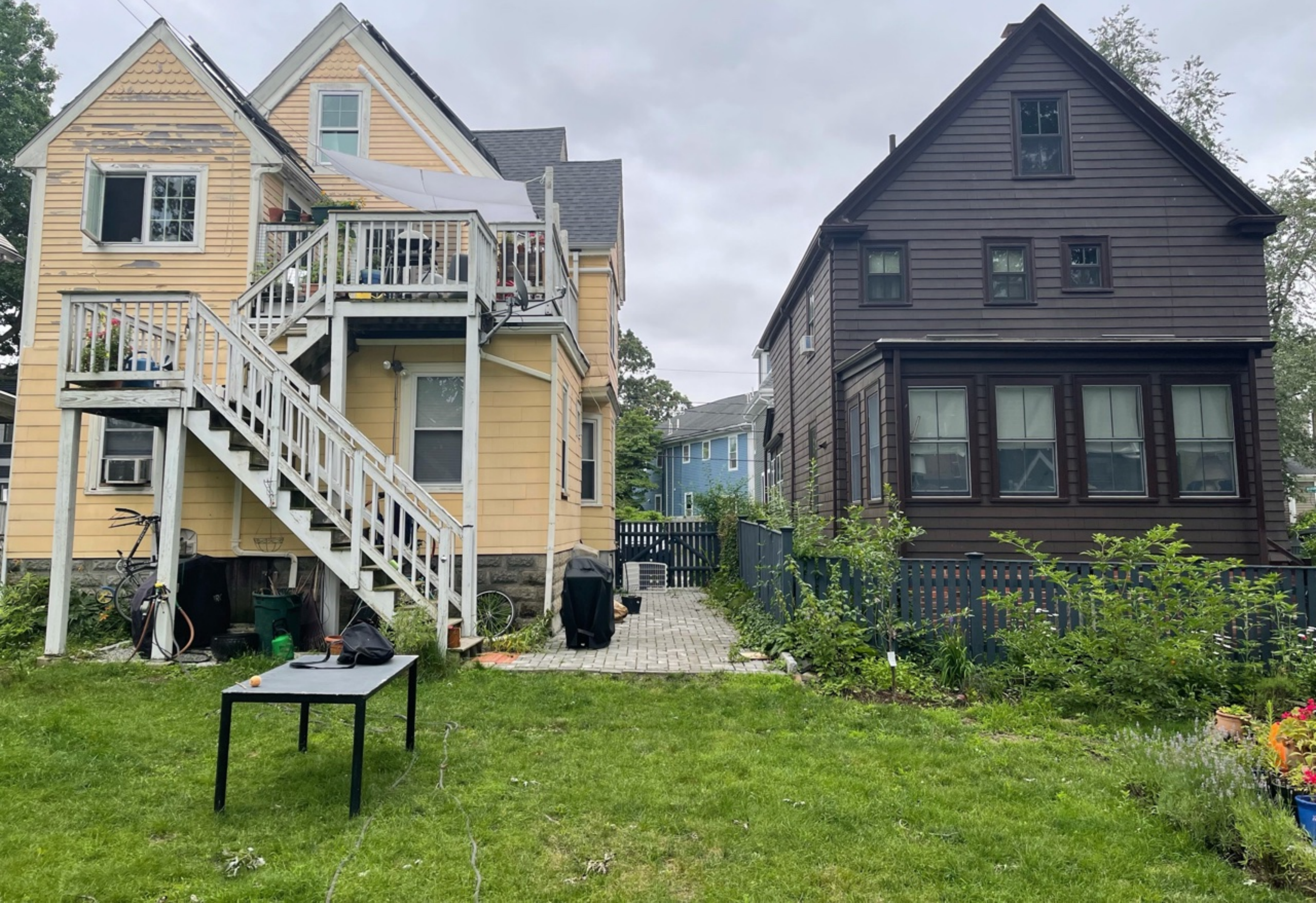
55 Washburn Avenue Rear View
