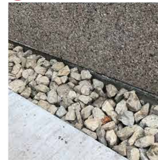
8 AGGREGATE DRIP STRIP
