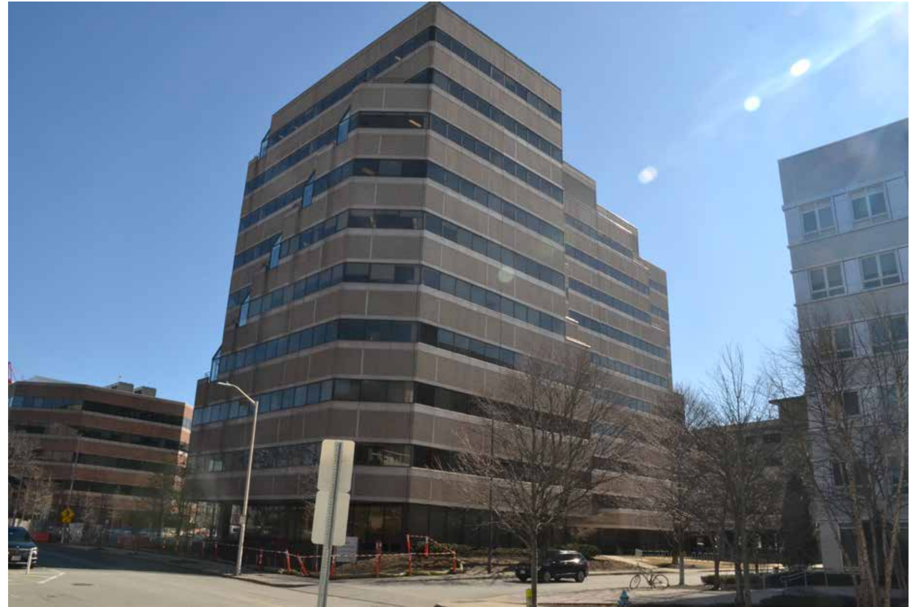
1 VIEW FROM CAMBRIDGE PARK DRIVE
