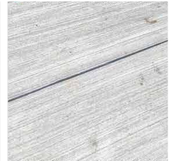
3 CITY STANDARD CONCRETE (SIDEWALK/ROW)
