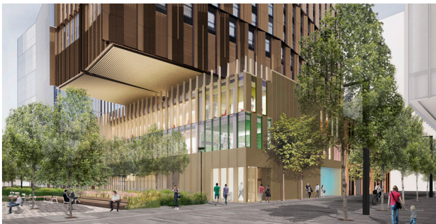
MIT has committed to building 950 additional graduate student beds, all of which will either be completed, under construction, or permitted by 2020. MIT's first project under this commitment (architectural rendering pictured) is under construction as of 2018.
