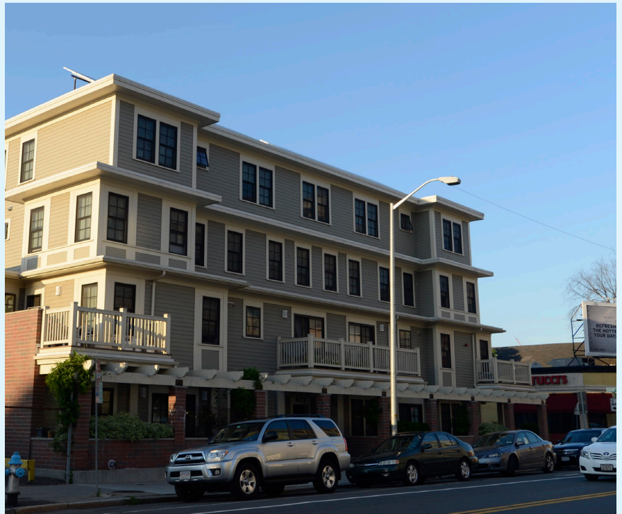
The City has facilitated the development and sale of hundreds of dedicated affordable homeownership units, including those at 821–825 Main Street (pictured).
