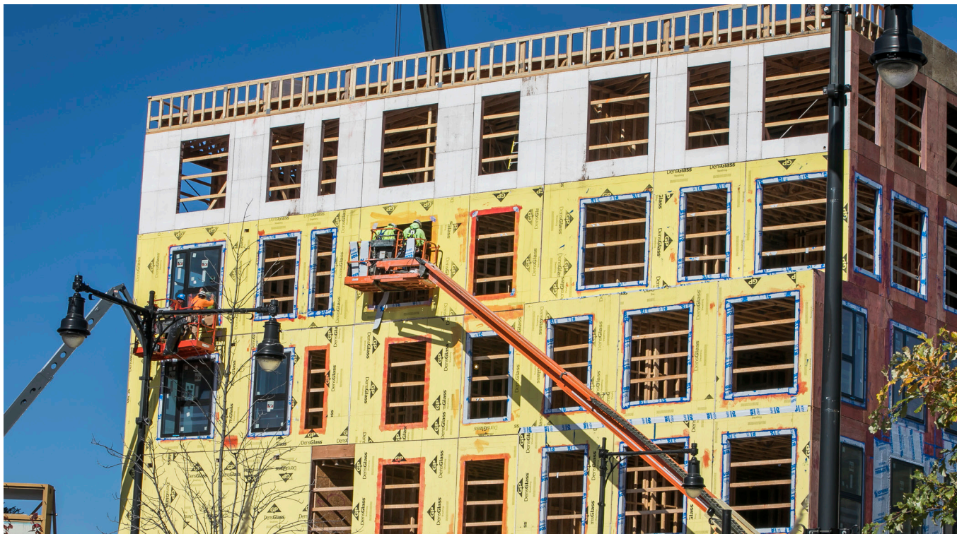
Construction in Cambridge in fall 2018.
