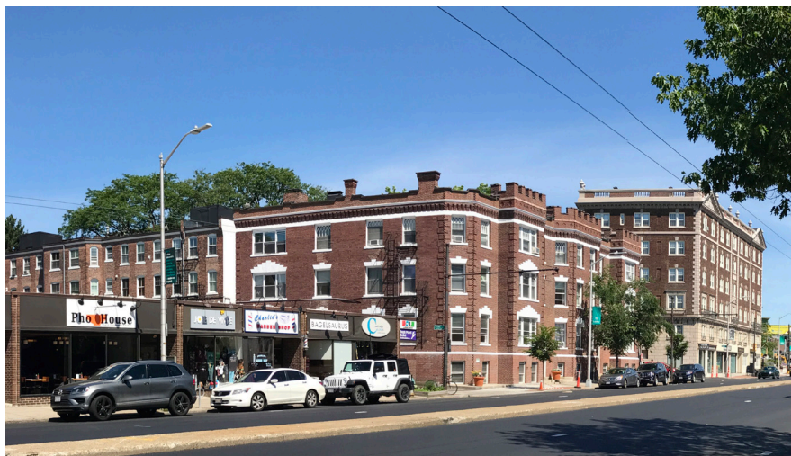
A mix of building densities on Massachusetts Avenue near Porter Square.
