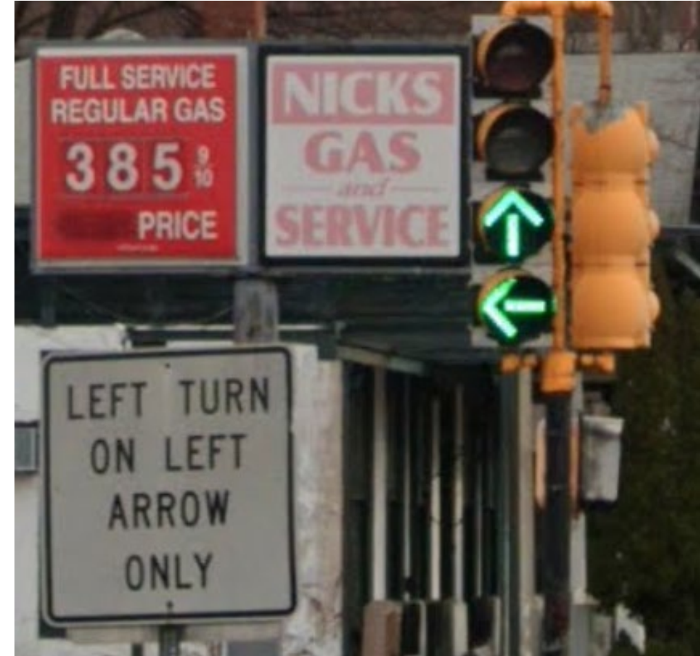
The existing signal equipment is side mounted rather than overhead and relies on supplemental signage for left turns
