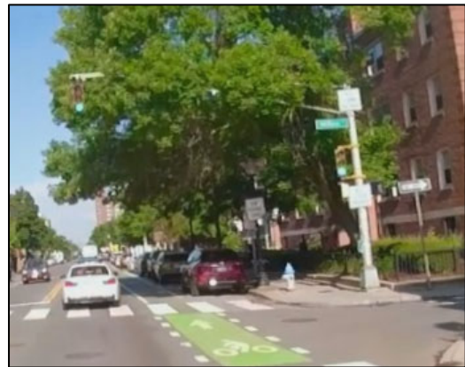
Image 6: Westbound signal head is difficult to see due to overgrown foliage, lack of backplates, and signal head size.
