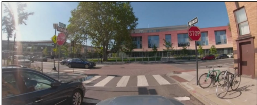
Image 7: The Hunting Street southbound approach has limited sight distance looking right due to a building on the northwest corner of the intersection.
