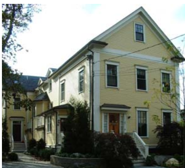
Figure 14. 25 Avon Street (1862), as renovated in 2003-05.
