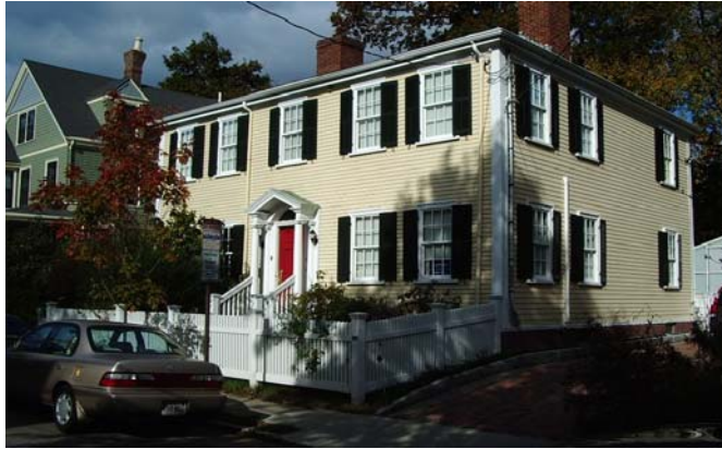
Figure 8. 26 Gray Street (1815, moved from Massachusetts Avenue in 1845).
