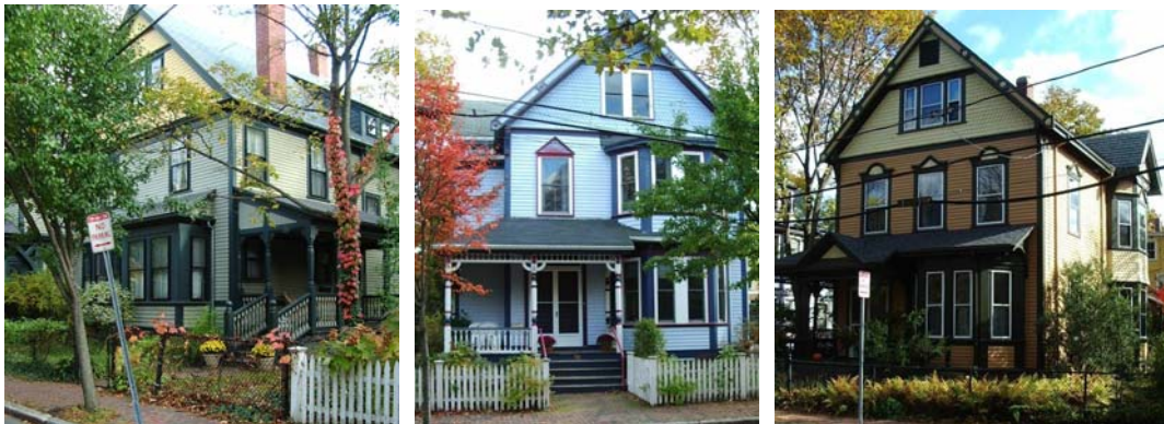
Figure 15. 14-16 Martin Street (1885, renovated and porch restored, 1998).
