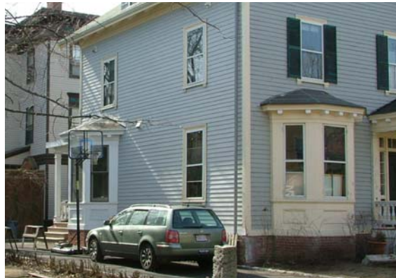
Figure 20. “The most conservative approach to planning an appropriate alteration is to ensure that it is exactly the same architectural style as the existing structure.” Bay window addition, 21 Bowdoin Street, (new bay at left; original at right, 2004-05).
