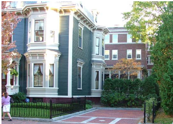
Figure 18. “Additions should defer to the original building; that is, they should be smaller than the original house, and should not draw attention away from it.” Addition (behind driveway), 24 Linnaean Street, 1998.
