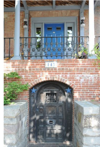
Basement entrance and front door
