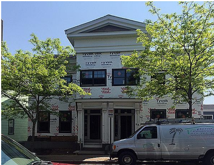
During construction, before stop-work order
