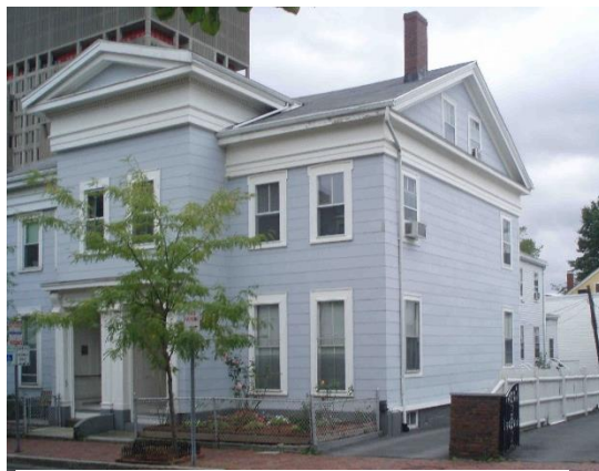
66-68 Otis Street, 2015 Assessor's photo
