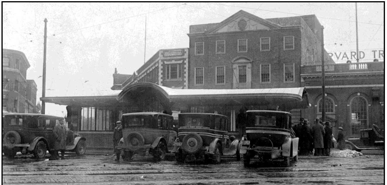
Harvard Station on completion, February 1928. This view shows the transparency desired by the proponents, already obscured by a taxi rank.
