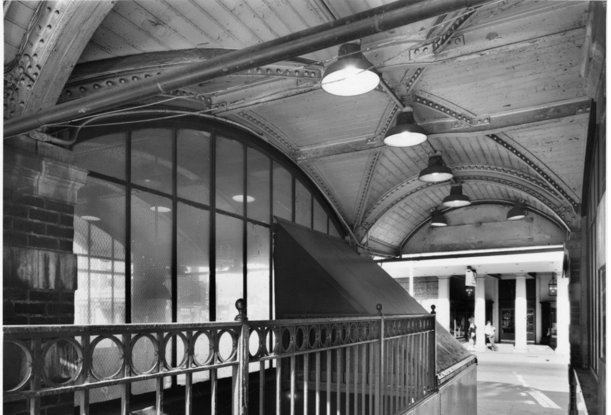
Passageway looking west, 1977
