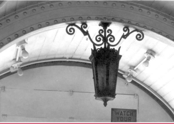
Lamp in passageway, ca. 1954-58. Bichajian photo
