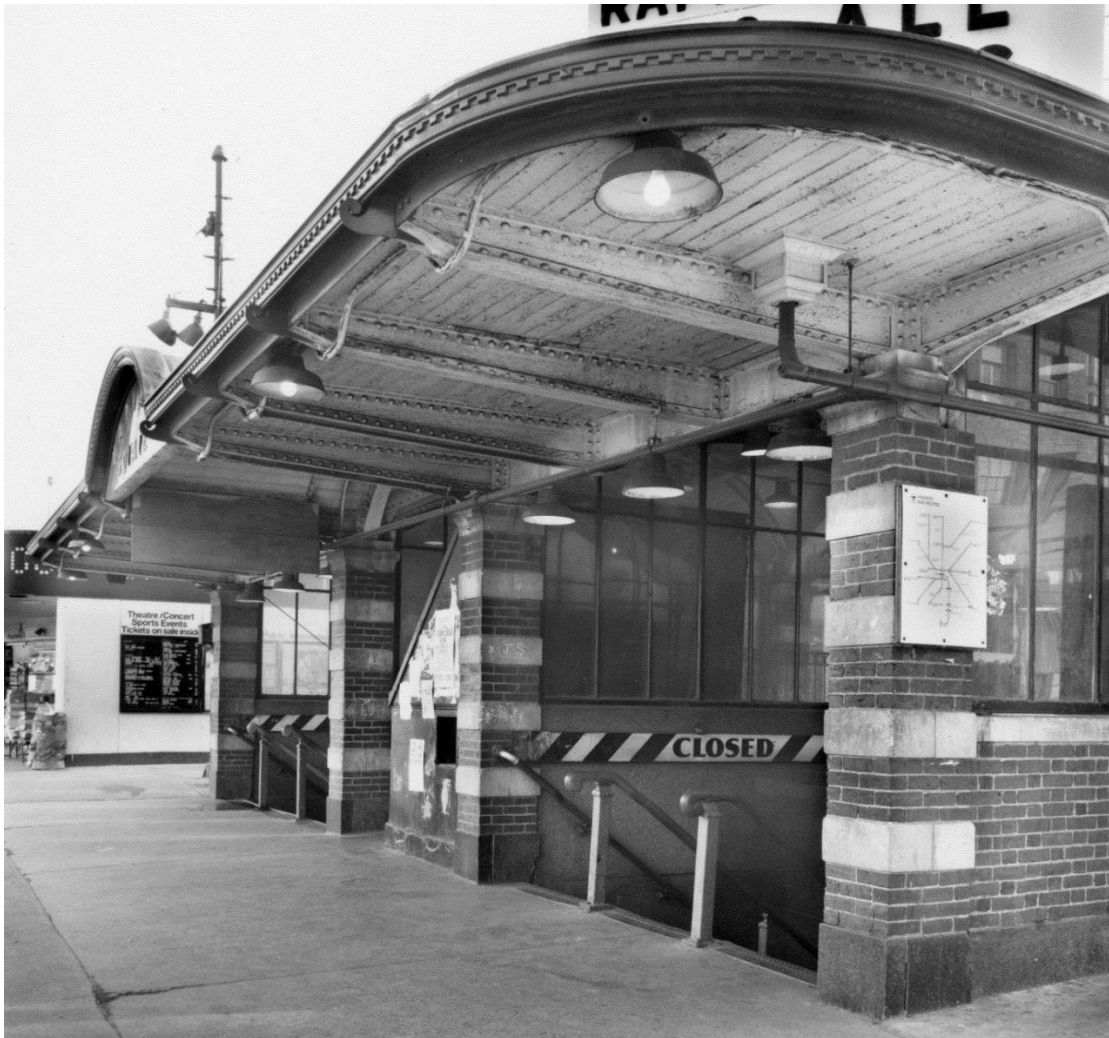
West elevation, 1977, showing roof edge dentil detail
