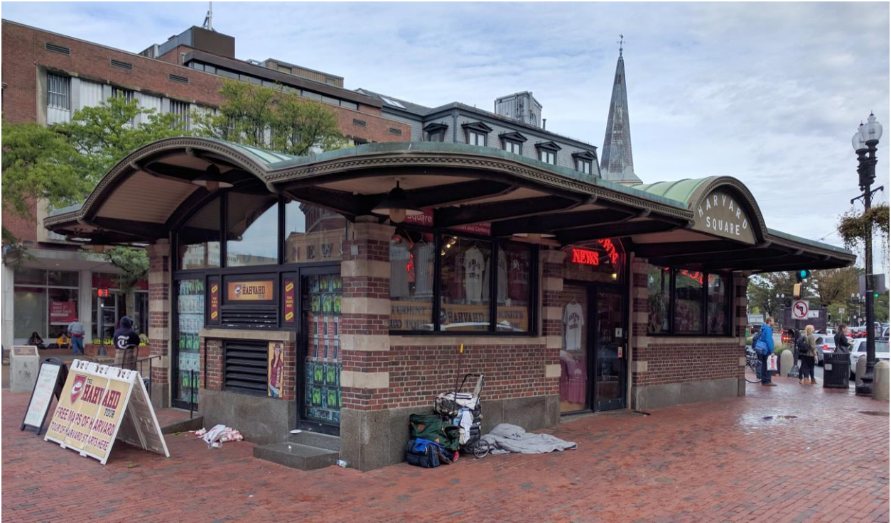
South and east elevations, 2016
