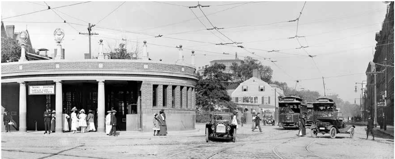
Harvard Square in 1912. The new headhouse was initially considered to be an ornament to the Square, but the design was hazardous to pedestrians and converging automobiles and streetcars. Library of Congress
