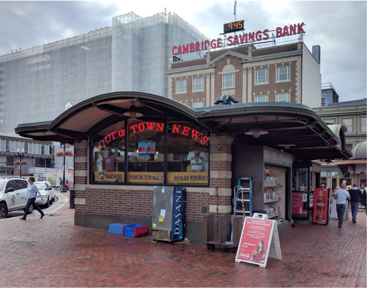
North and west elevations, 2016
