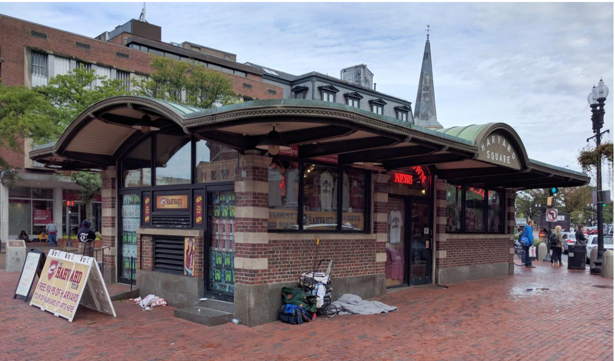
South and east elevations, 2016
