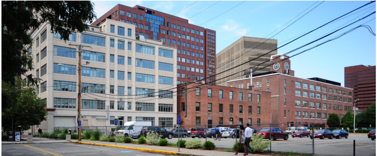
Suffolk, Hammett, and Kendall Square buildings, south elevations. CHC photo, July 2012
