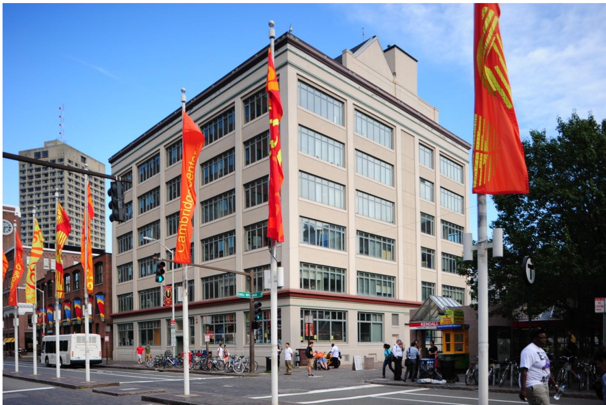
Suffolk Engraving & Electrotyping Building, 292 Main Street. CHC photo, July 2012
