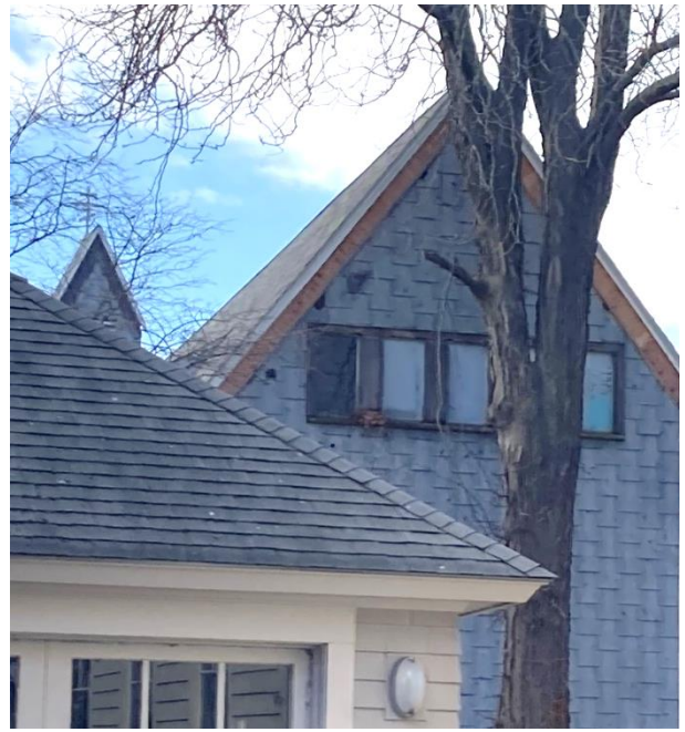
Figure 98 Chancel windows on rear façade. CHC.
