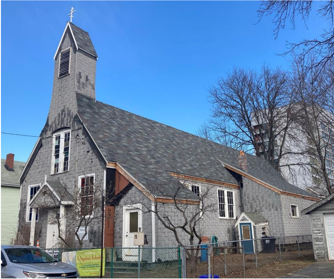
Figure 6 View of St. Augustine's African Orthodox Church front and east façades with new roof. CHC.
