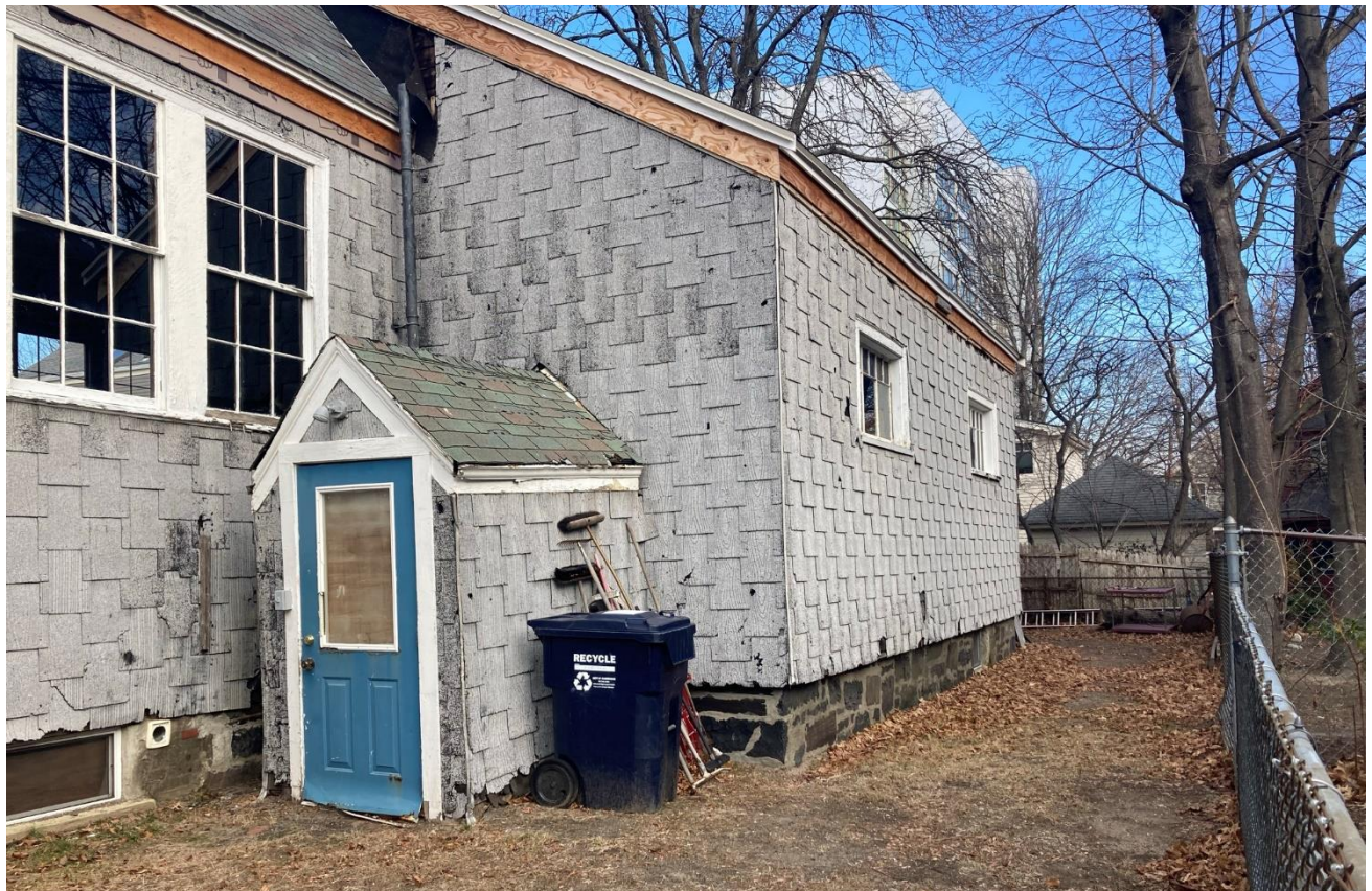
Figure 10 Non-original bulkhead entry. CHC
