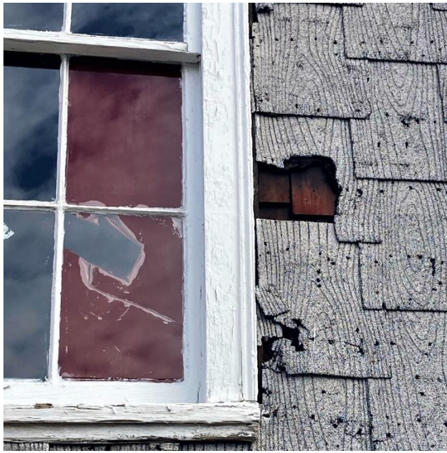
Figure 8 Asphalt siding with exposed original cedar shingles. CHC
