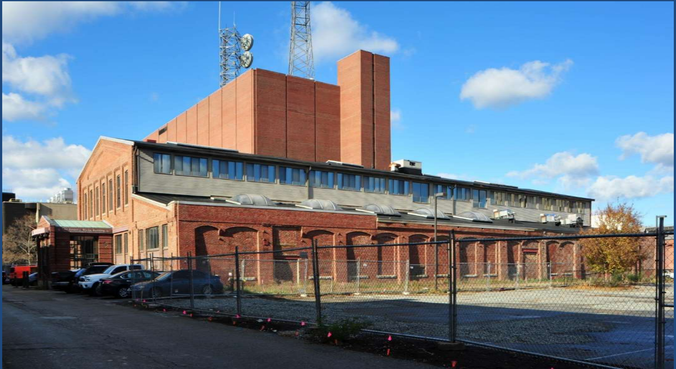
South and east elevations
