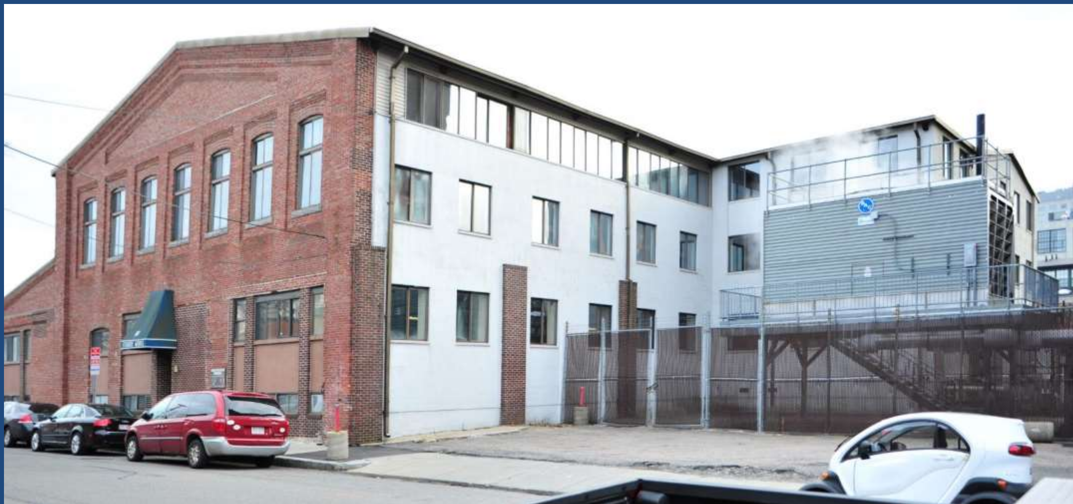
North and west elevations, showing removed portion of original building
