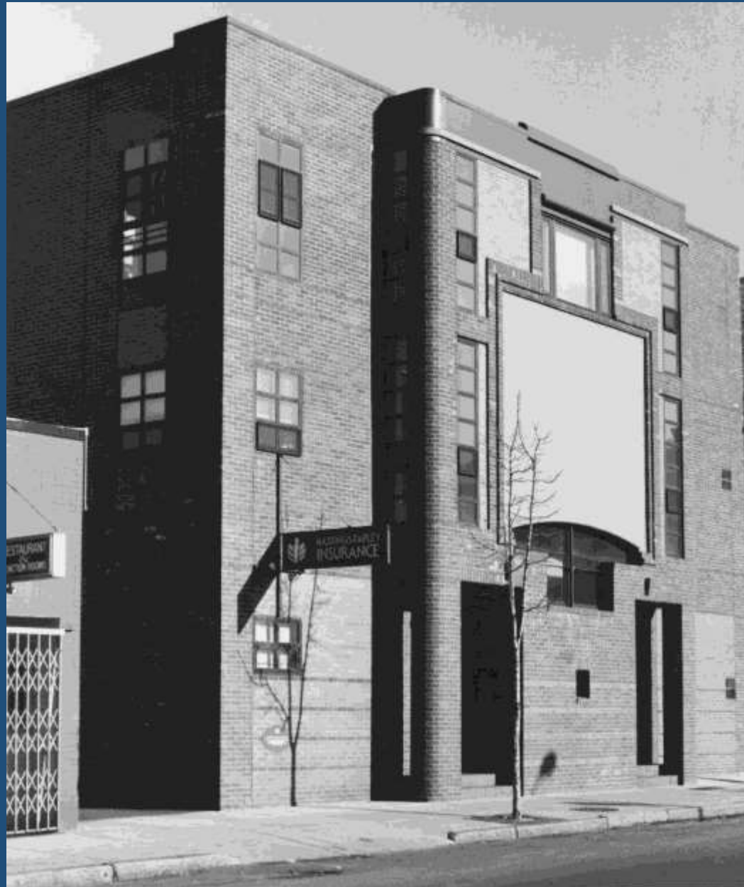
Two floors added above 1969 original (1983, Fred Koetter Associates, architects). Photo 1985
