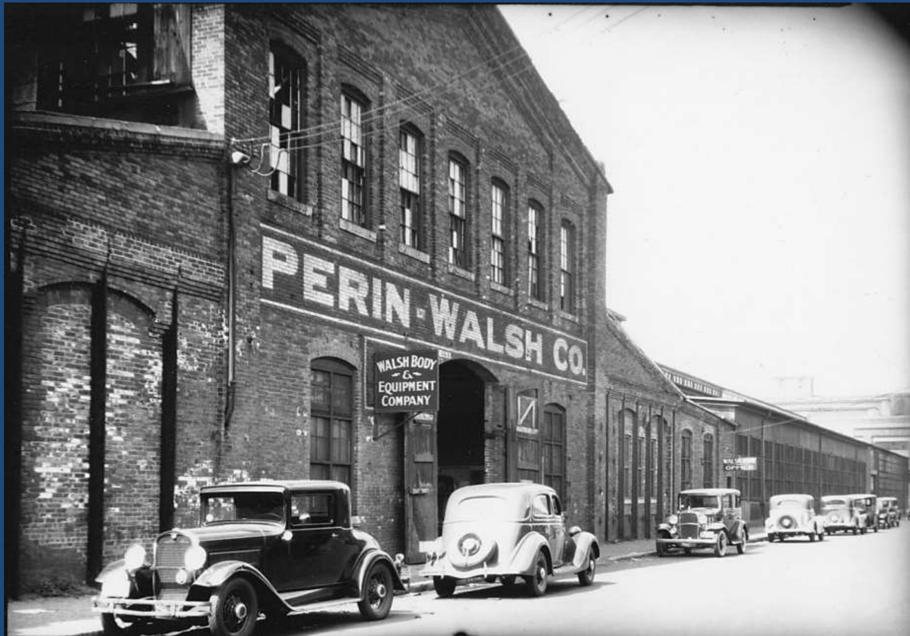
Bent Street (north) elevation, ca. 1936
