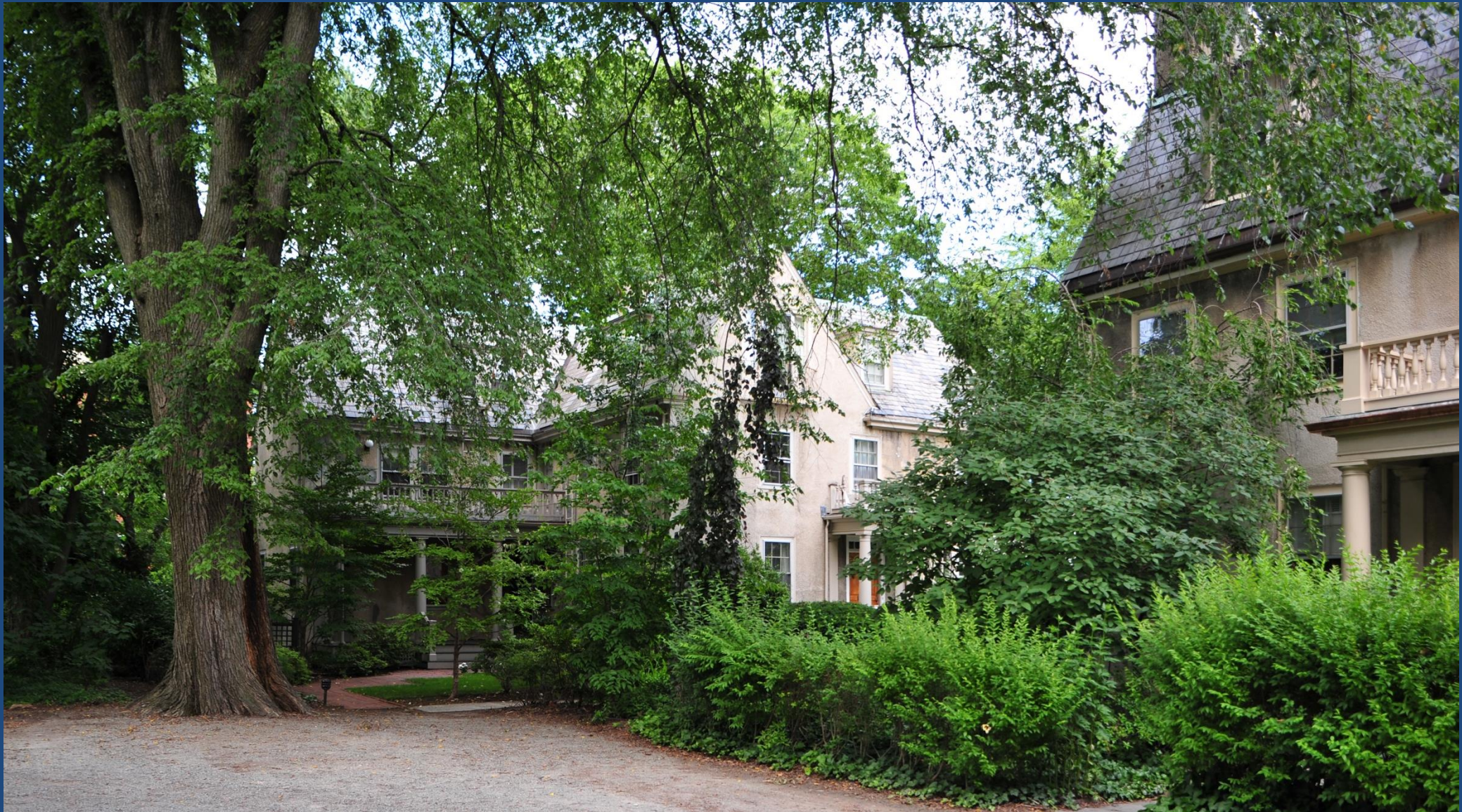
9 Shady Hill Square (1915, J.W. Ames, architect)
