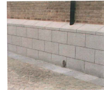
⑥ REJUVENATED EXISTING RED BRICK WALL
