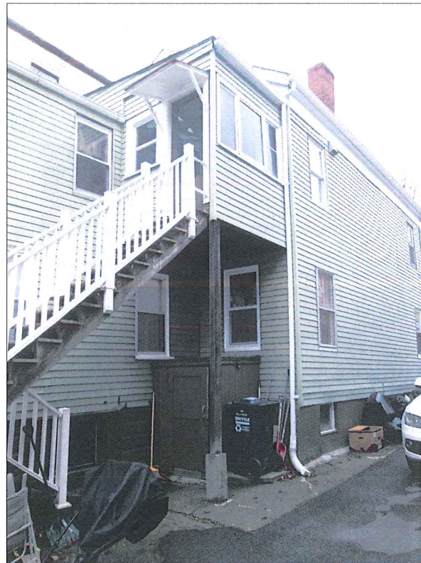
5 REAR CORNER AT STAIRS
