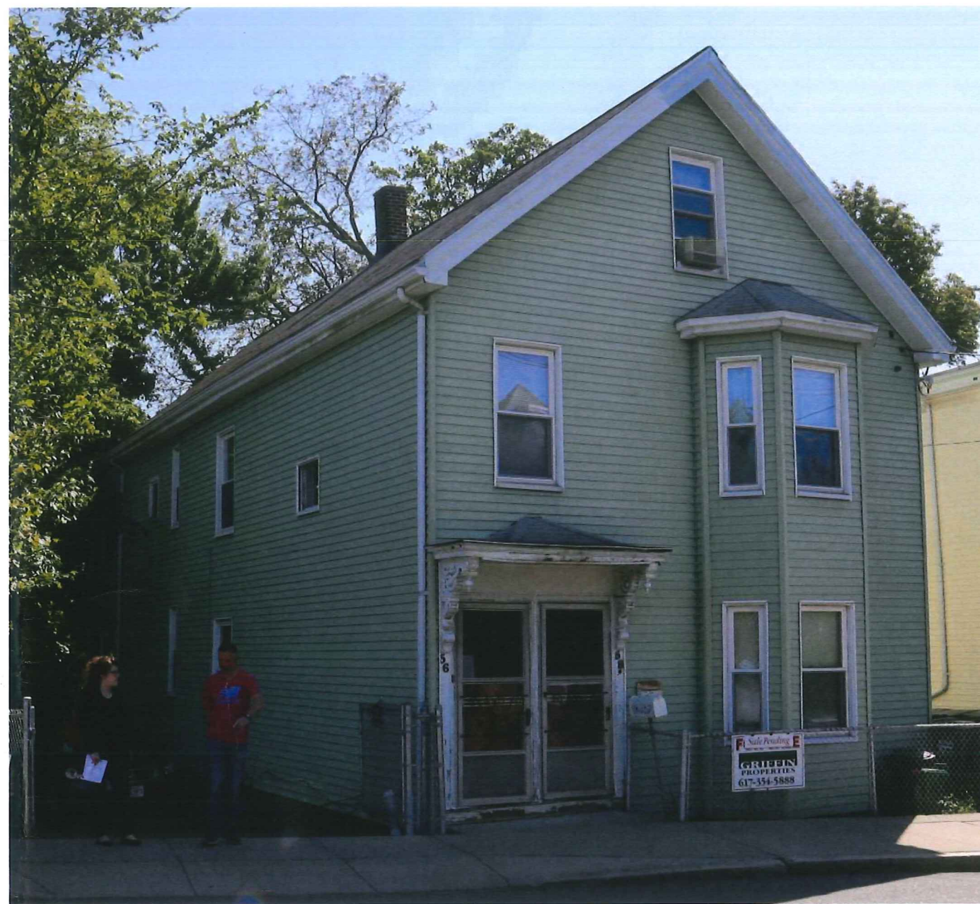
56 WALDEN STREET - FRONT/LEFT VIEW
