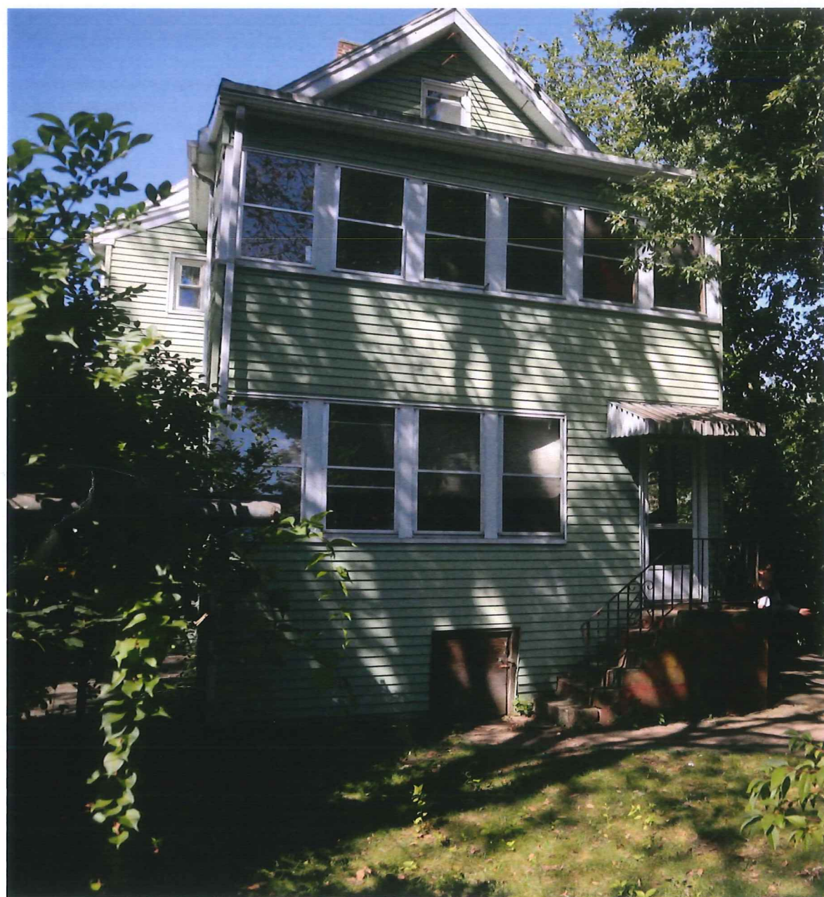
56 WALDEN STREET - REAR VIEW
