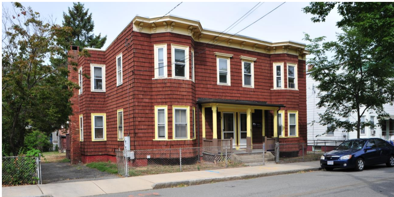
54-56 Reed Street, demolished 2016. 60-62 Reed Street is at right
