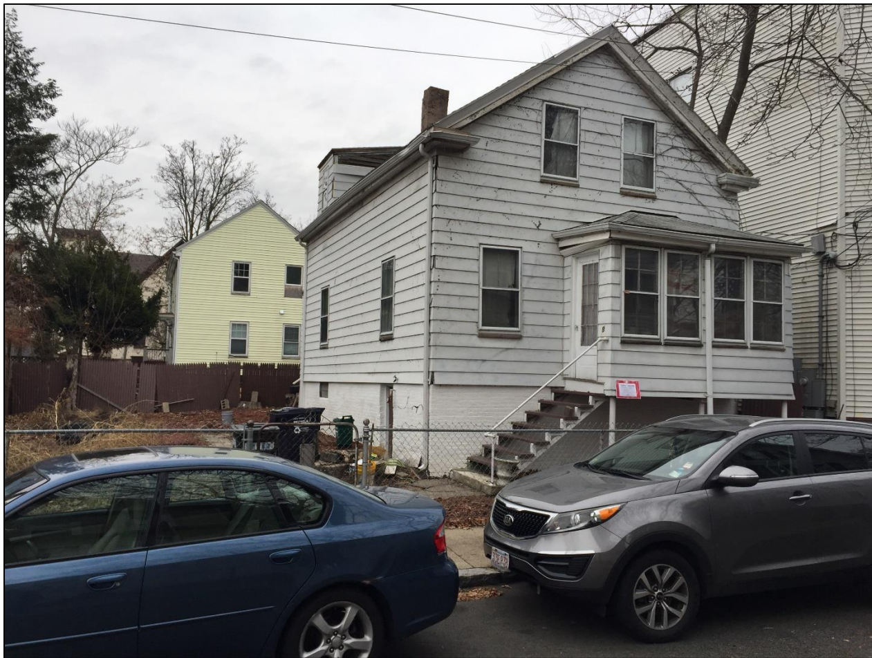
9 Pine Street, front (east) elevation with enclosed porch addition
