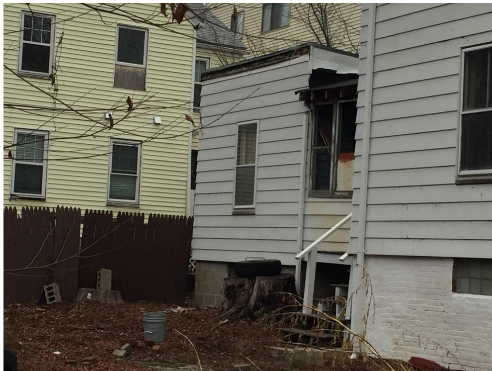
9 Pine Street, south side of the ell and 1886 rear addition, 2019
