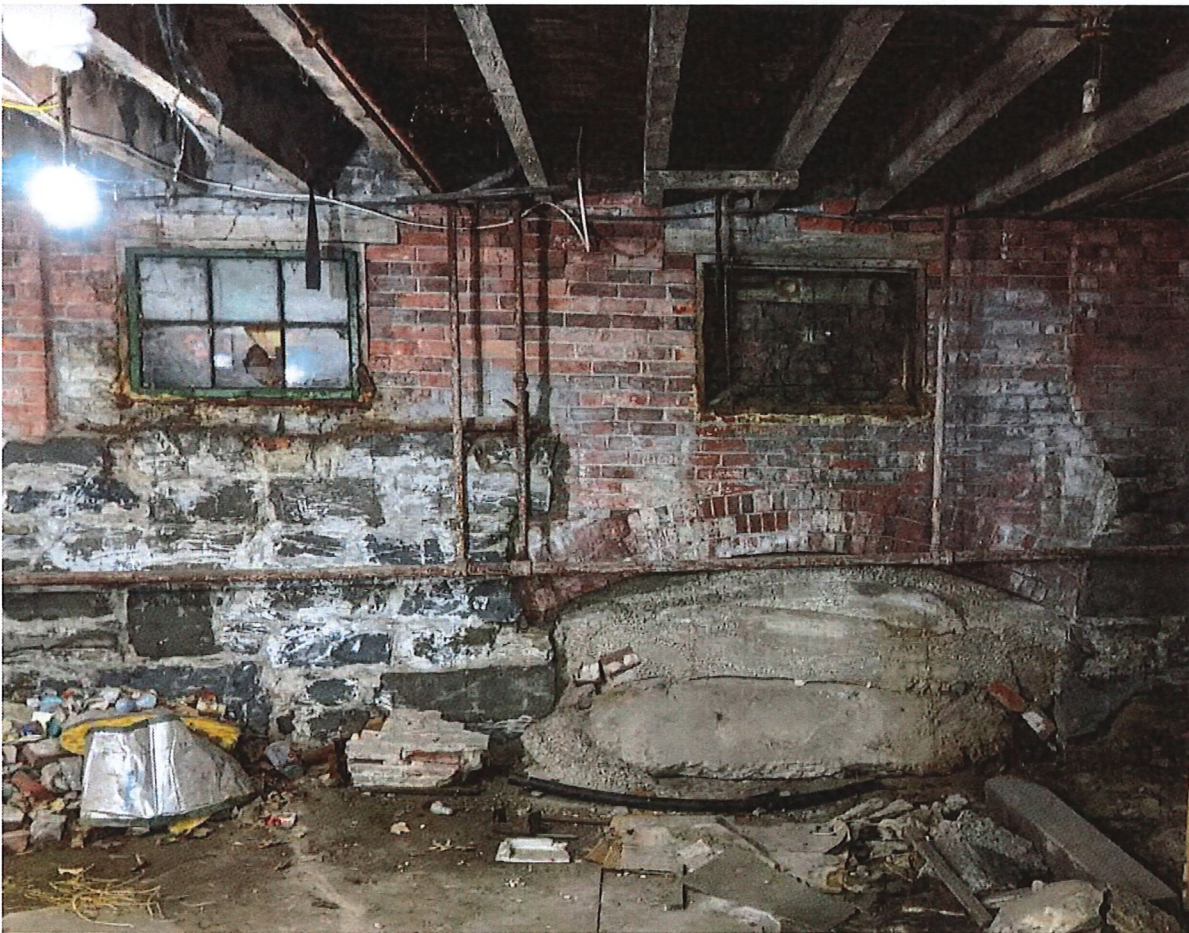
West foundation, showing brick relieving arch filled with concrete, July 16, 2020.
