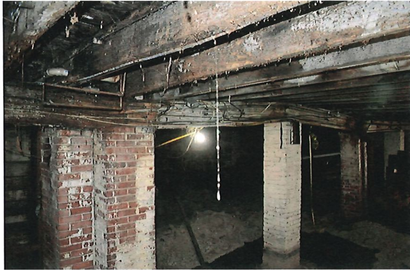
Figure 10 Central beam in basement
