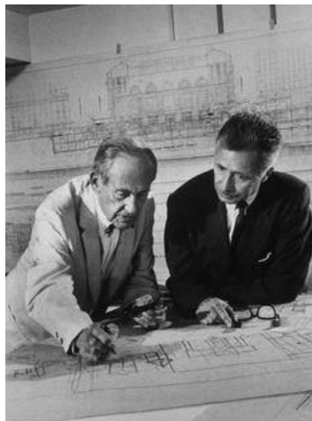
Walter Gropius and Pietro Belluschi at work on the Pan Am Building
