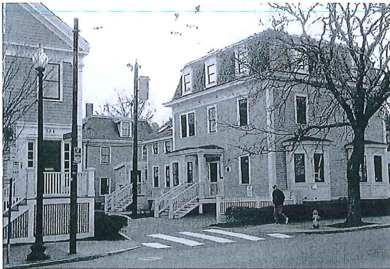
HCM-323: 138 Mt. Auburn Street, by Loreda, LLC. Alter exterior, demolish rear ell, and construct new ell.
