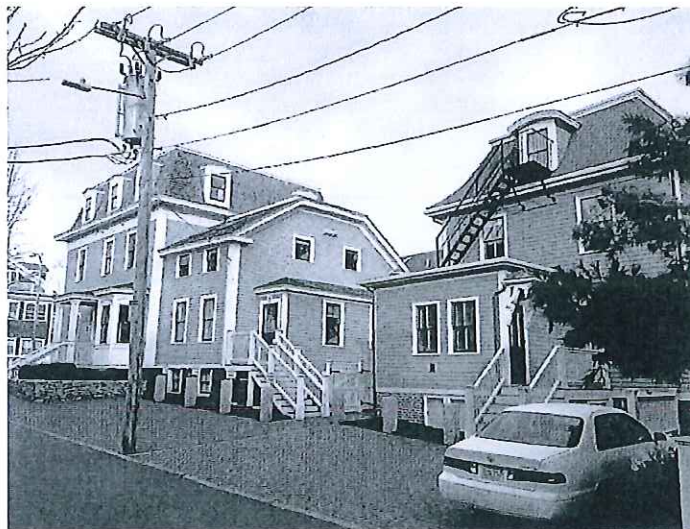
HCM-323: 138 Mt. Auburn Street, by Loreda, LLC. Alter exterior, demolish rear ell, and construct new ell.
