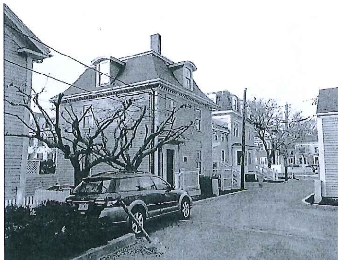
HCM-323: 138 Mt. Auburn Street, by Loreda, LLC. Alter exterior, demolish rear ell, and construct new ell.
