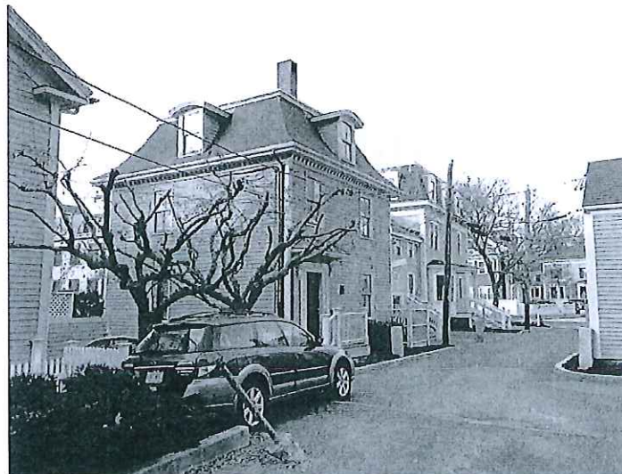
HCM-323: 138 Mt. Auburn Street, by Loreda, LLC. Alter exterior, demolish rear ell, and construct new ell.
