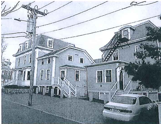
HCM-323: 138 Mt. Auburn Street, by Loreda, LLC. Alter exterior, demolish rear ell, and construct new ell.
