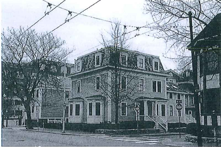
HCM-323: 138 Mt. Auburn Street, by Loreda, LLC. Alter exterior, demolish rear ell, and construct new ell.
