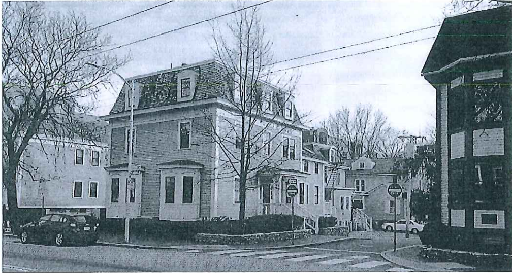
HCM-323: 138 Mt. Auburn Street, by Loreda, LLC. Alter exterior, demolish rear ell, and construct new ell.
