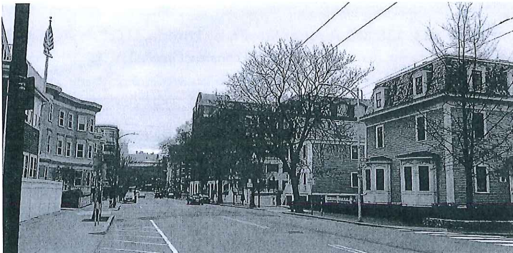
HCM-323: 138 Mt. Auburn Street, by Loreda, LLC. Alter exterior, demolish rear ell, and construct new ell.
