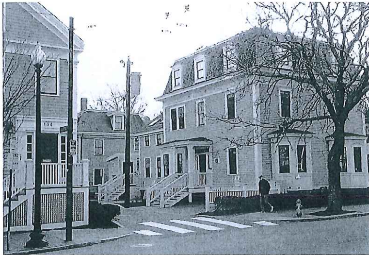
HCM-323: 138 Mt. Auburn Street, by Loreda, LLC. Alter exterior, demolish rear ell, and construct new ell.
