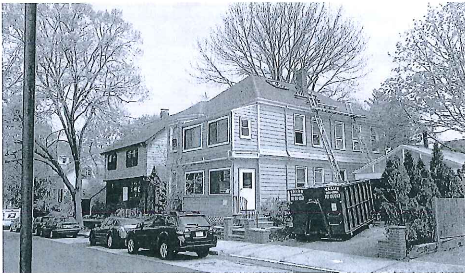
HCM-335: 7-9 Gibson Street Alter windows and demolish chimney
