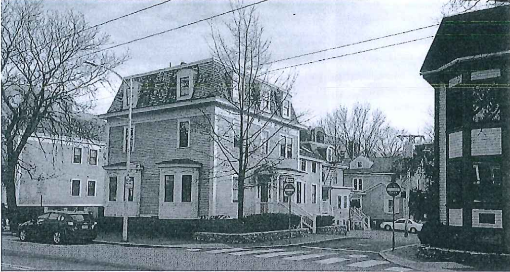
HCM-323: 138 Mt. Auburn Street, by Loreda, LLC. Alter exterior, demolish rear ell, and construct new ell.
