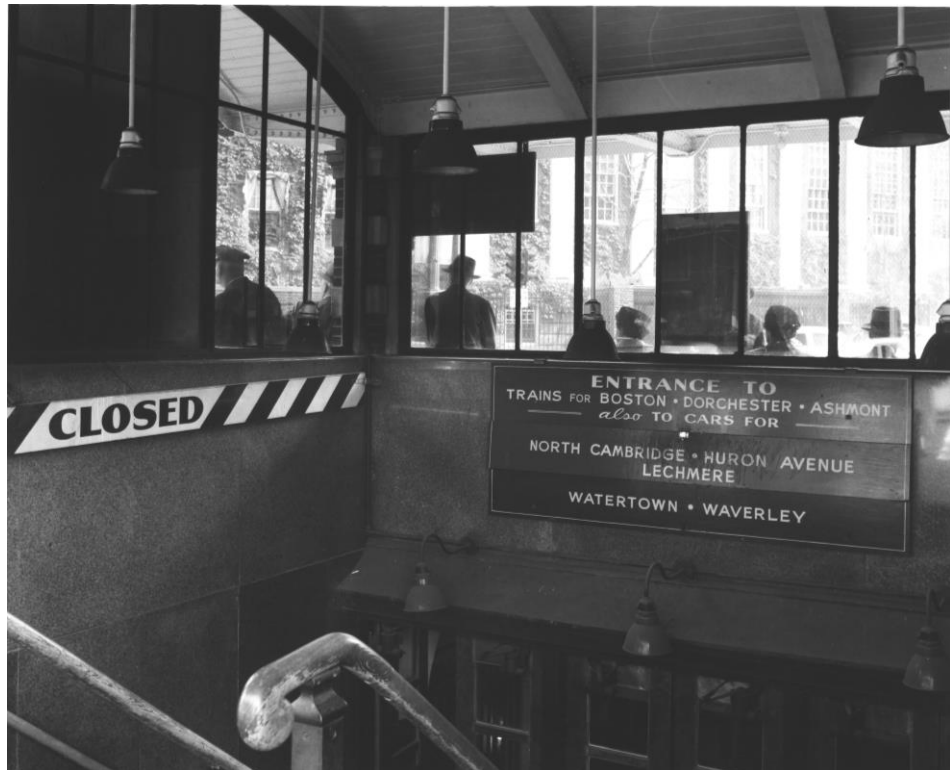
Entrance (north) stairway, ca. 1954-58
