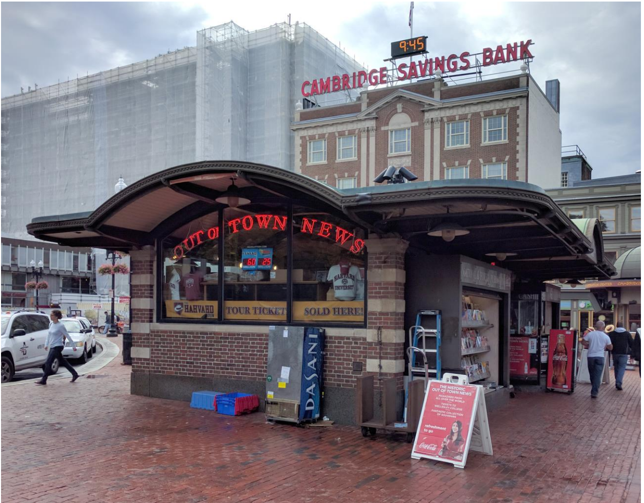
North and west elevations, 2016, showing pendant light fixtures installed in 1990
