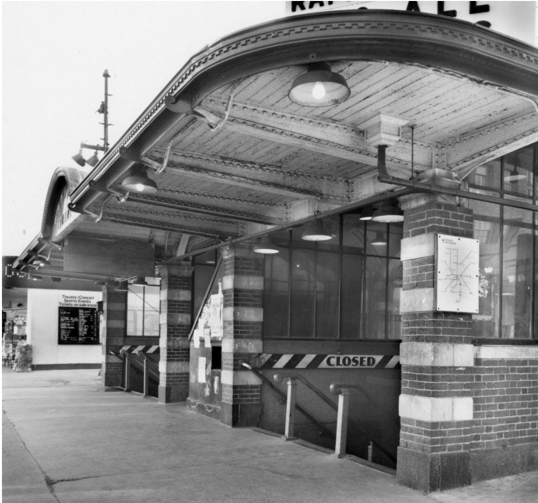
West elevation, 1977, showing roof edge dentil detail
