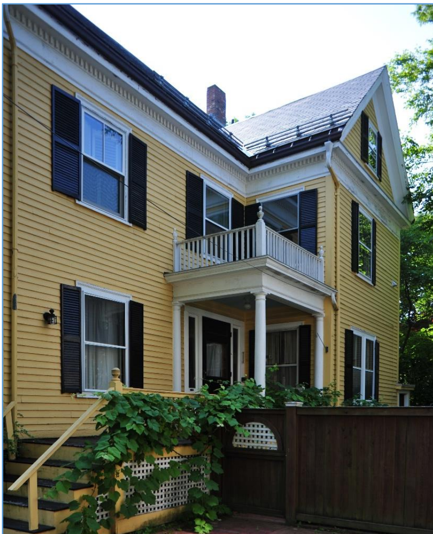
25 Walker Street, front door and porch detail CHC photo
