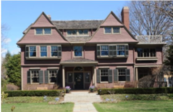
113 Brattle St. (1887, Andrews, Jaques & Rantoul, architects)
