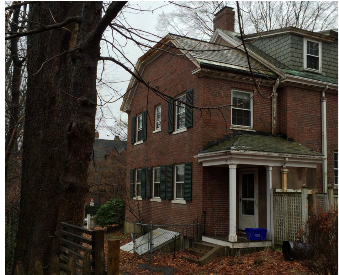
EAST ELEVATION (NE corner)
