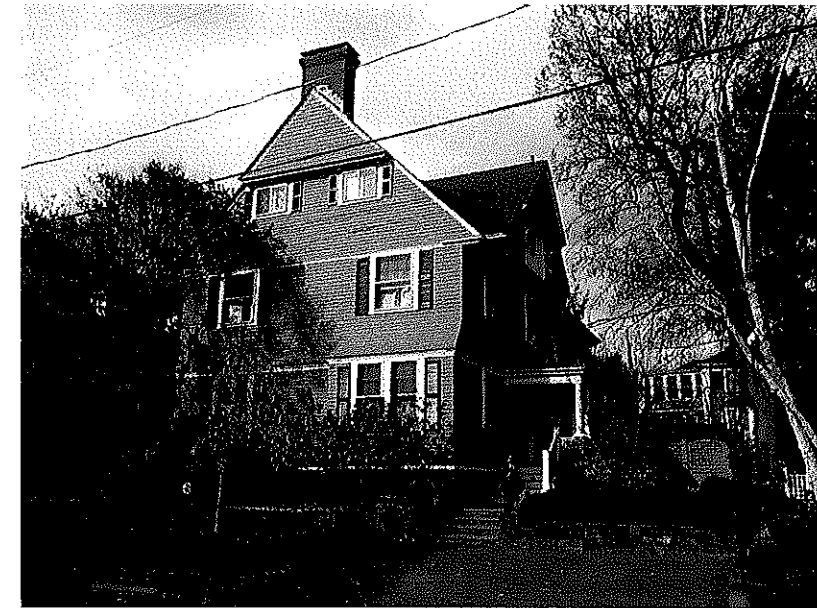
⑥ VIEW OF EXISTING FRONT ELEVATION
